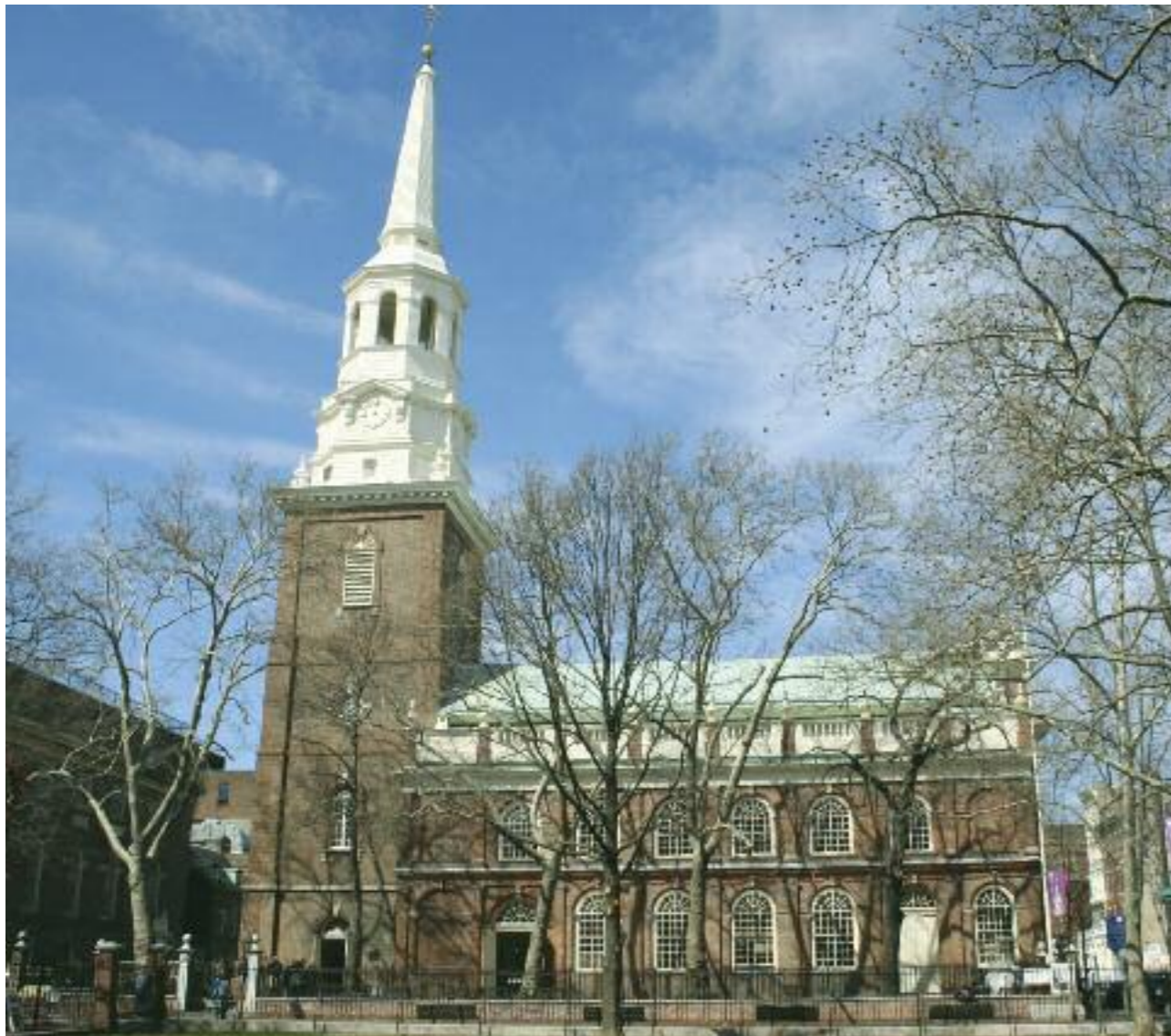
Christ Church in Philadelphia, USA, built in the 1700s with a copper roof.
