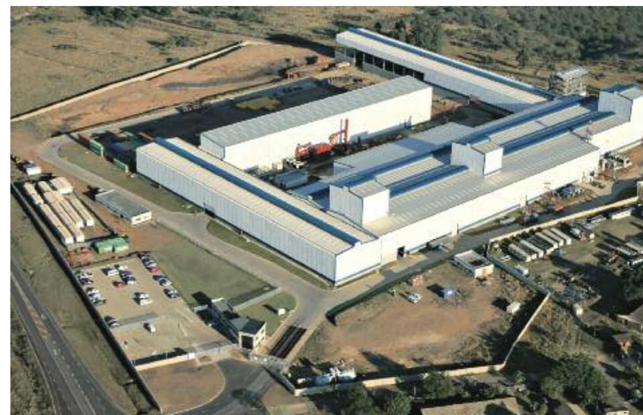
Safal Steel coil coating complex in KwaZulu-Natal, South Africa.
