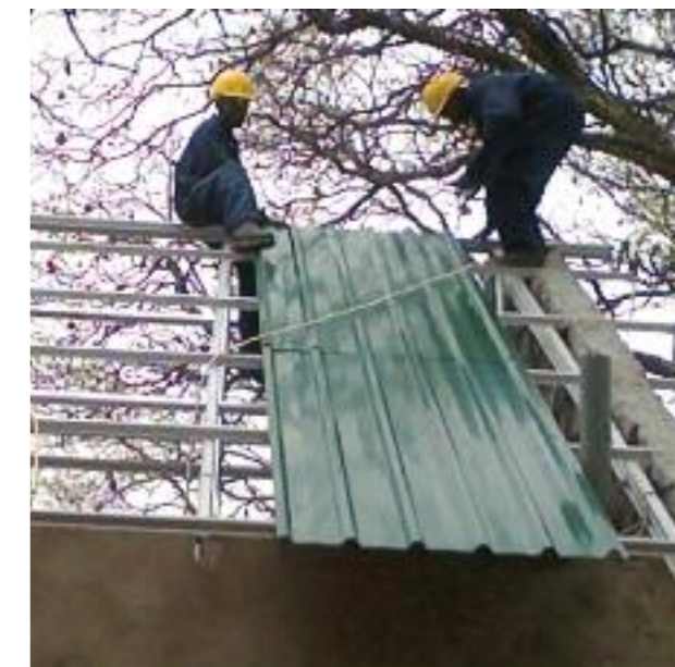
Affordable housing under construction.
