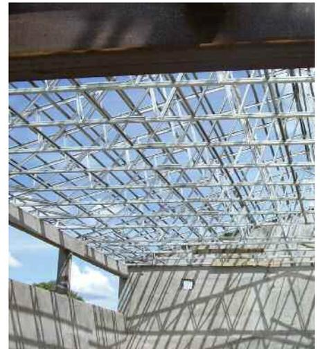
Ultraspan is a light gauge steel truss system, supported by patented software known as MiTek 20/20, which minimises design time and maximises productivity.
